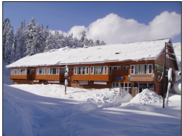
ADHOC SUB CENTRE, GULMARG
